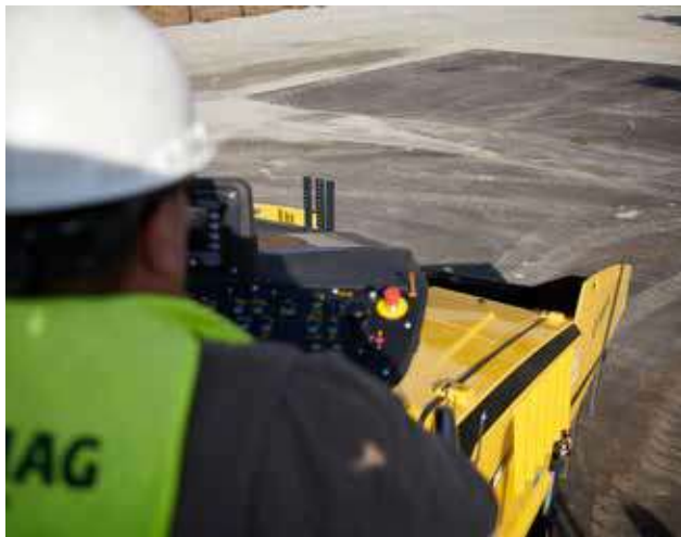
Improved line of sight to hopper ...
